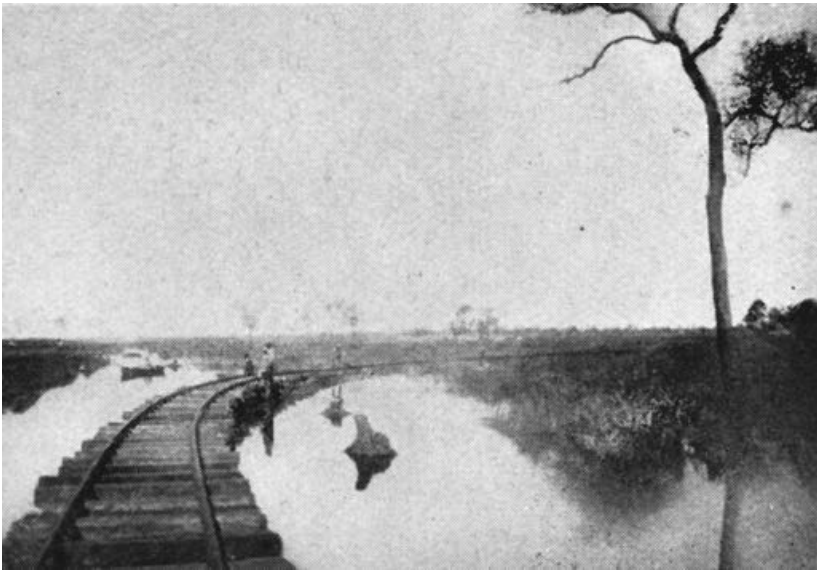
Rail construction in the Pantanal, 1910s. Reprinted from Cardoso Ayala and Simon, Album Graphico do Estado de Matto-Grosso, 155.
